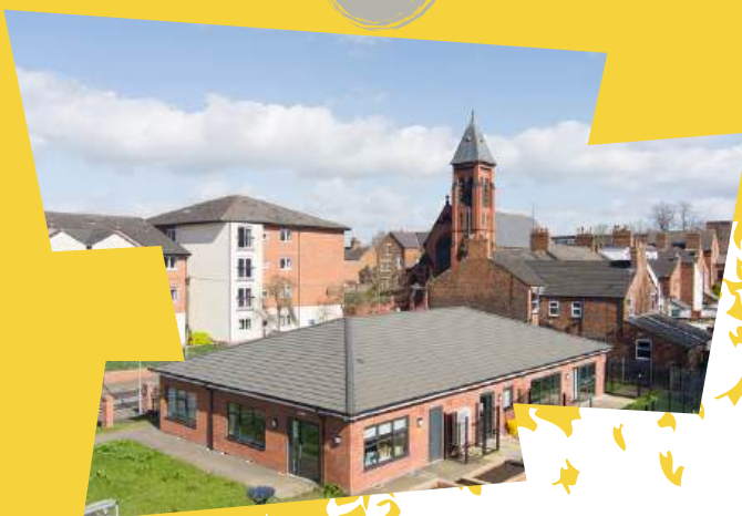
Aerial view of the St. Mary's Caritas Centre, Crewe.
